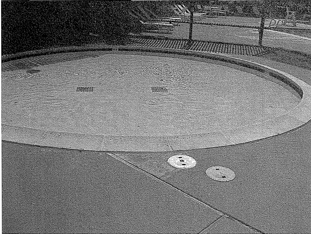
EXHIBIT 6: NO DECK DEPTH MARKERS
