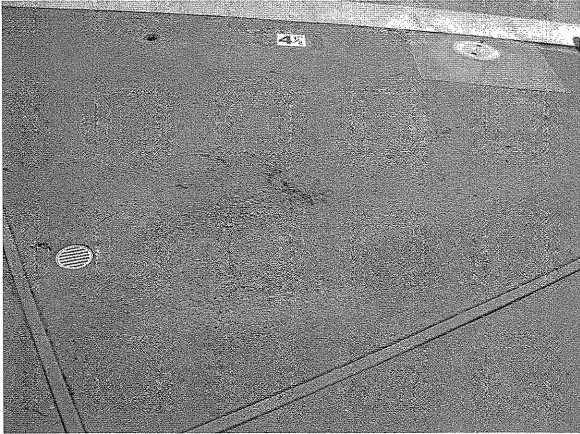
EXHIBIT 10: EXISTING POOL DECK
